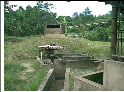
A Biogas Digestion Unit at a Pig Farm But could be used on a zero grazed dairy farm
